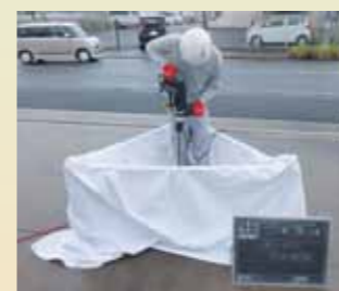
①土間削孔状
